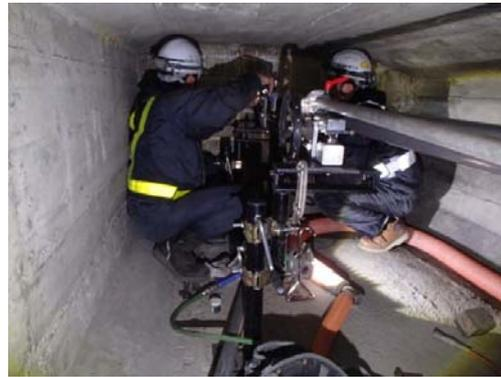
Photo 4. Water jet drilling
