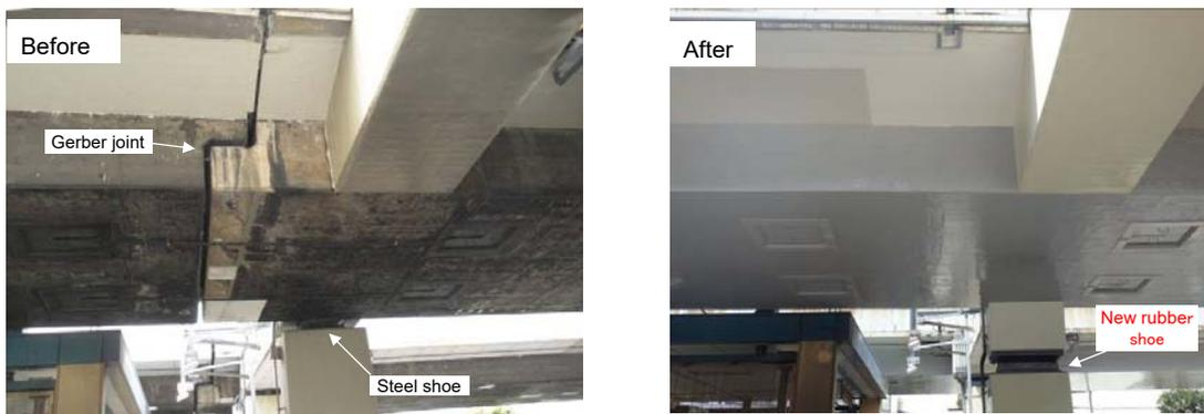
Photo 5. Gerber joints made continuous
