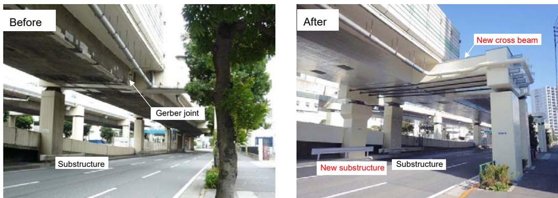
Photo 6. Gerber joints separated with new substructure
